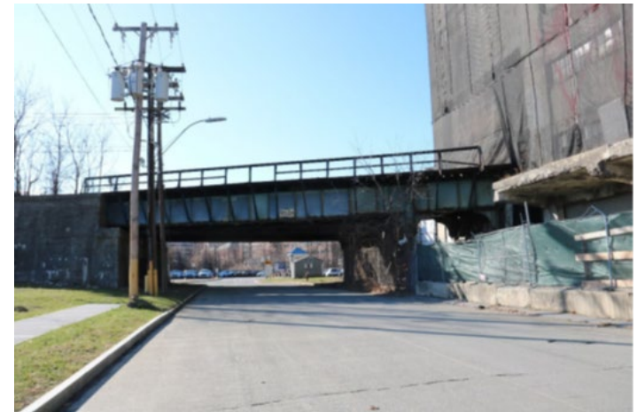
Bridge and Rail Spur Entering the Second Floor of the Central Warehouse
