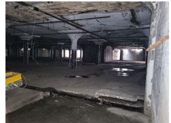
Abatement Complete. 11 th Floor
