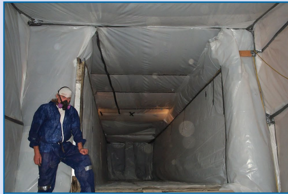
POLY LINED TRUCK FOR ACM TRANSPORTATION
