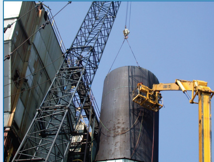
RIGGING AND HOISTING
