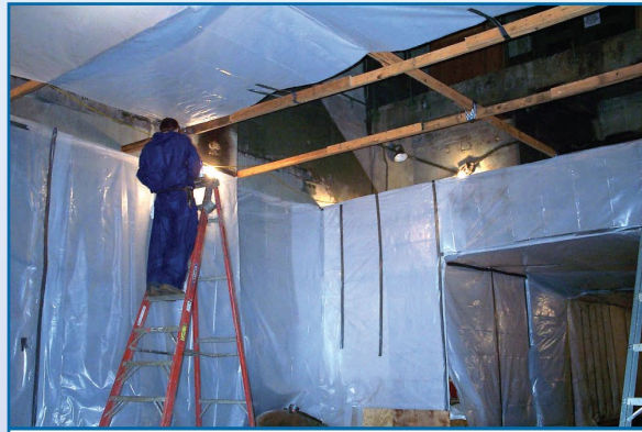
WORK AREA PREPARATION
