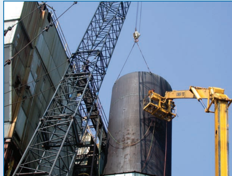
RIGGING AND HOISTING
