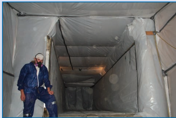
POLY LINED TRUCK FOR ACM TRANSPORTATION
