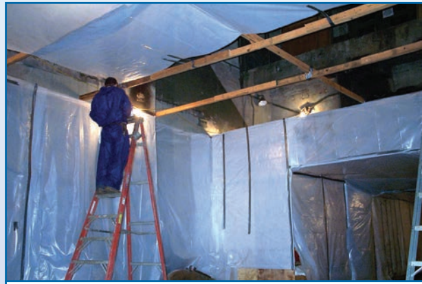
WORK AREA PREPARATION
